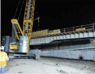
The I-238 team designed a falsework cover that integrated into the bridge girders themselves and the contractor re-sequenced the work. This new design not only protected the BART tracks and allowed enough vertical clearance, but also had a number of advantages:
