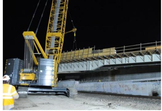
*Kent Bridge pre-assembled girders suspended by crane pick (Photo – Flatiron West, Inc.)*
